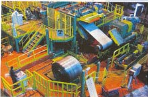
Figure 4. Uncoiling and entry looping section
