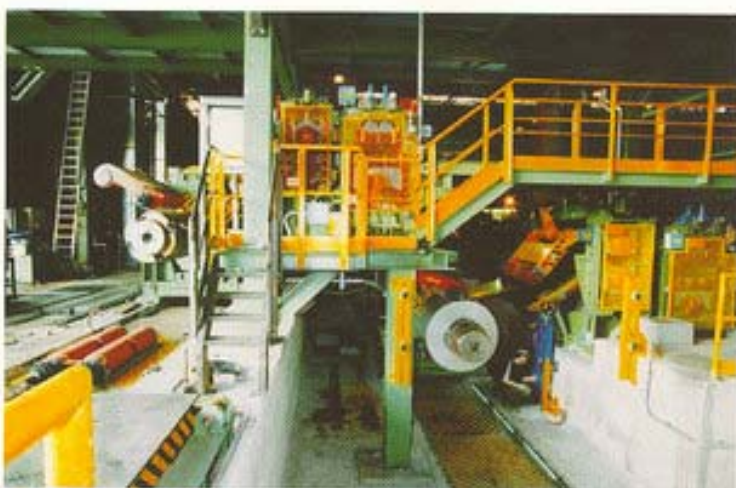
Figure 1. Uncoupling and entry section (TK AST Terni)
