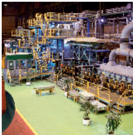
Fig 5 Tin dissolution plant at Ternium Siderar
